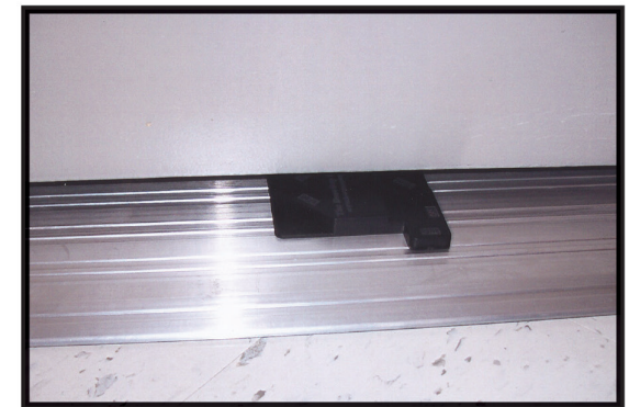
Bottom of Door with Sill With Raised Noncombustible Sill
